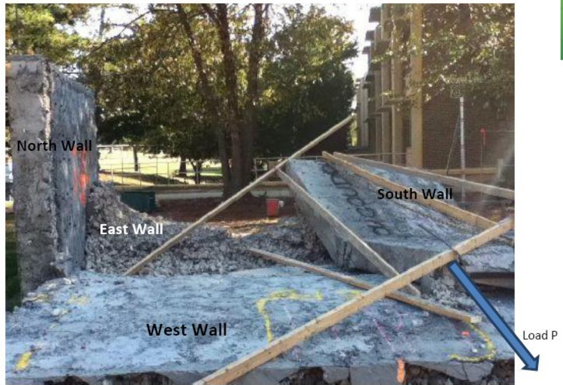
(a) Rubble-House after failure
