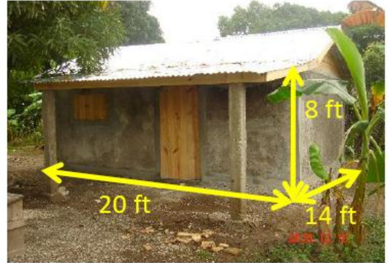
(g) Final look of a typical Rubble-House in Haiti
