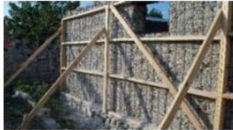
(c) Baskets filled with loose rubble
