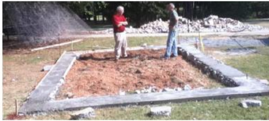
(a) Foundation installation
