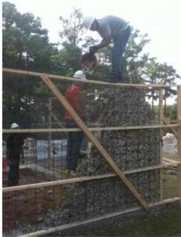
(c) Wire baskets being filled with loose rubble.
