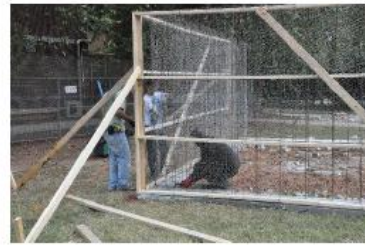
(b) Wire basket installation
