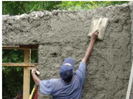
(e) Applying cement finish
