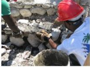
(a) Foundation installation
