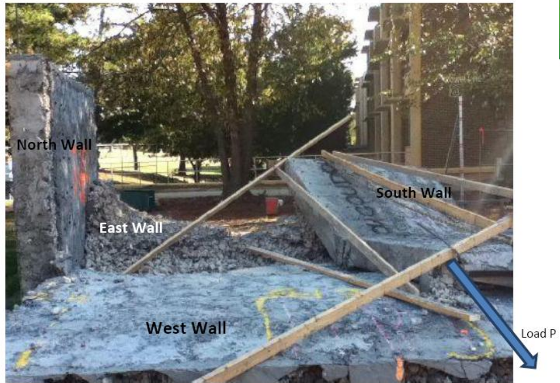
(a) Rubble-House after failure
