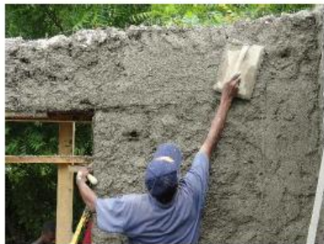
(e) Applying cement finish
