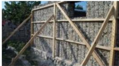
(c) Baskets filled with loose rubble
