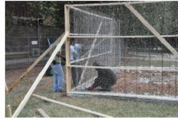
(b) Wire basket installation
