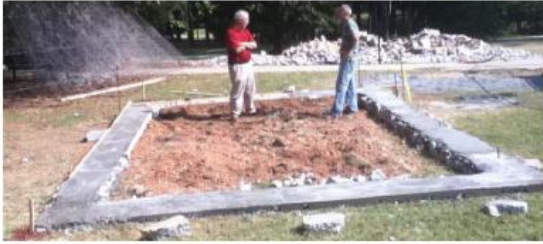
(a) Foundation installation
