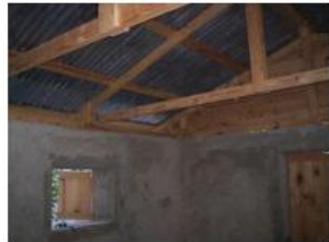
(f) Roof installation
