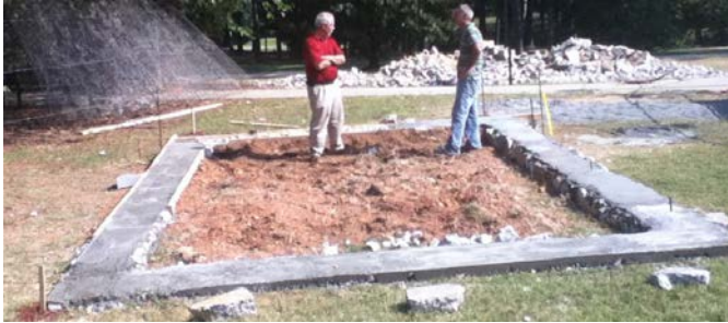
(a) Foundation installation
