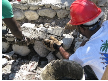
(a) Foundation installation
