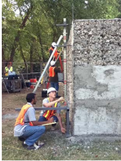
(a) Displacement gauges
