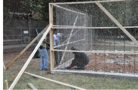
(b) Wire basket installation
