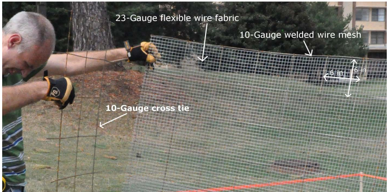
Figure 2 Preparation of the wire basket.
