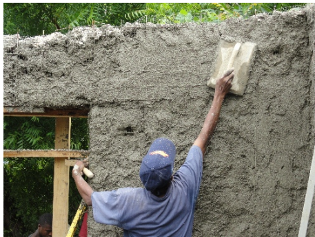
(e) Applying cement finish
