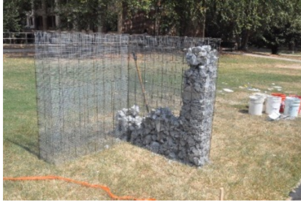
(a) Demo Wall partially filled with rubble.
