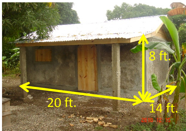
(g) Final look of a typical Rubble-House in Haiti
