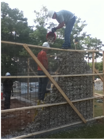
(c) Wire baskets being filled with loose rubble
