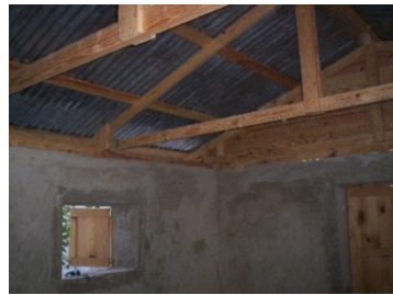
(f) Roof installation
