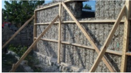
(c) Baskets filled with loose rubble
