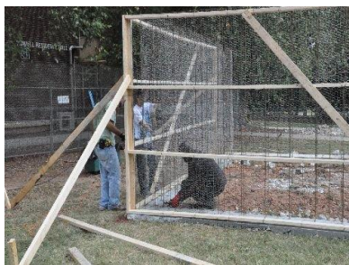
Stage 3: Wire basket erection
