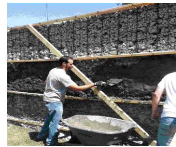
Stage 5: Finishing rubble walls
