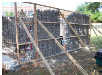
Stage 4: Pouring the rubble into the Basket
