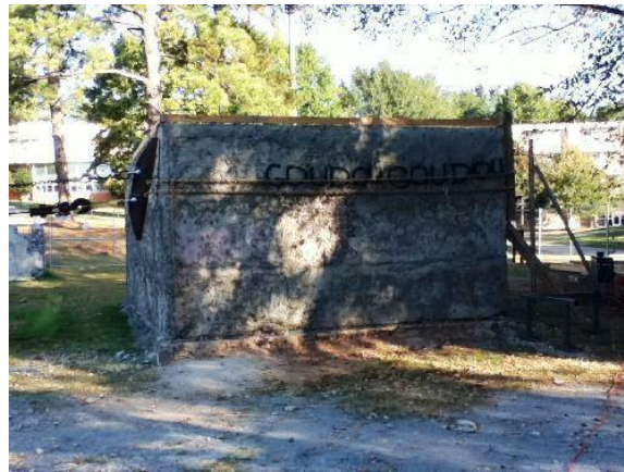
Test 3: Destructive Test (South Wall)
